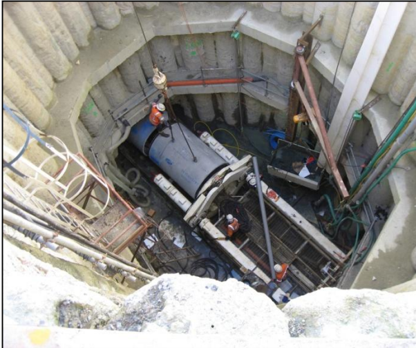
Photograph 6-4 Set up of pipe segment to be jacked into place
