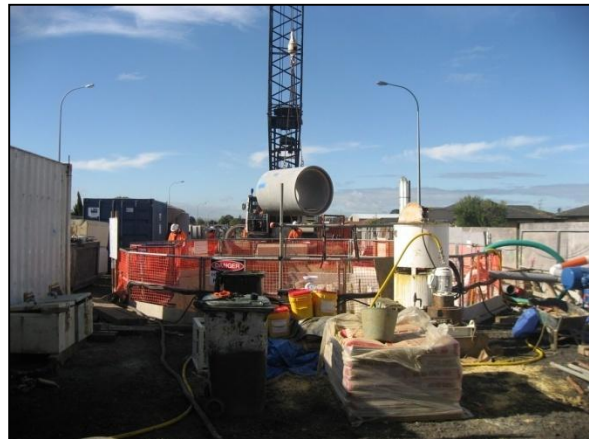
Photograph 6-3 Pipe segment being lowered into place by crane
