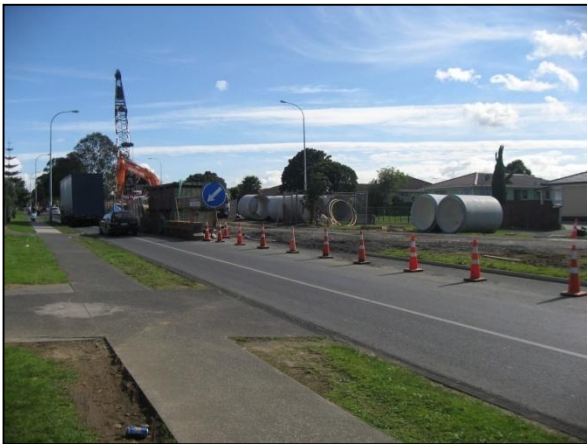
Photograph 6-2 View of construction (launch) site
